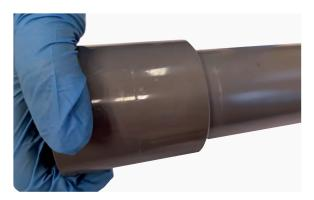
**Step 6** – Immediately after application of cement, push pipe fully home into fitting. Do not twist. Hold pipe & fitting for times varying from a few seconds on sizes 1/2", to 1 minute on sizes 5" and above. It is important to create the joint swiftly, to enable assembly without excessive force being required.
