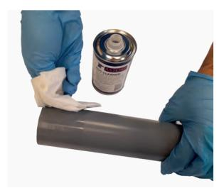
**Step 4** – Thoroughly clean the surface of the pipe length to be inserted using a clean, lint free cloth or paper towel, moistened with Astore Eco-cleaner.
