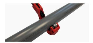
**Step 1** – Cut pipe to length using a rotary plastic pipe cutter as shown. Where possible clamp the pipe in a vice, avoiding excessive distortion. The pipe must be cut square. The use of a rotary pipe cutter is preferred over the use of a hacksaw as the finish is clean, leaving no loose swarf or burr on the pipe. If a saw is used, it is essential that all burrs and loose materials are removed.
