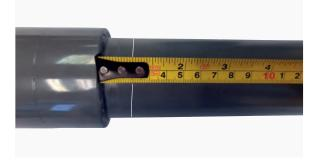
**Step 8** – Using measurement b (see point 3), check that the pipe has been fully inserted.
