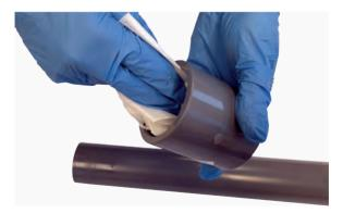
Repeat the cleaning process on the inside of the fitting.
