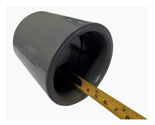
**Step 3** – Measure the insertion depth of the fitting. Make two marks on the pipe; a) the insertion depth b) 20mm longer than the insertion depth.
