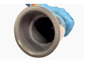
Application of correct amount of cement will result in a neat bead at edge of fitting & pipe. Excessive deposits inside fittings must be avoided as these can weaken the pipe wall, particularly on small sizes. When working in cold conditions, ensure joints are free from frost & moisture and allow extra curing time to compensate for lower temperatures.
